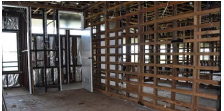
Demolition works in progress.
